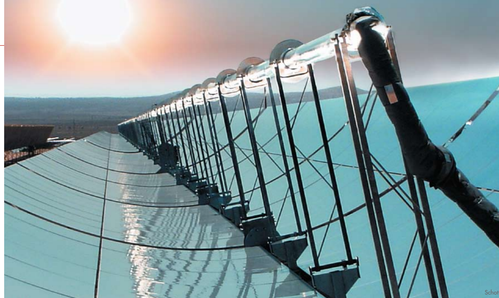
The parabolic trough collectors are up to 400 m long and track the sun's radiation. The thermal oil in the central receiver pipe transports the received energy to the power station unit.
